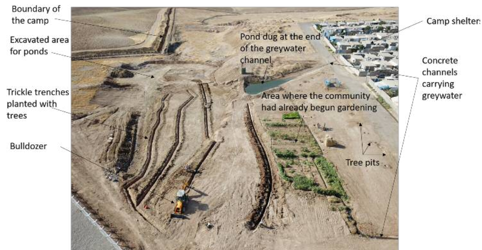
Fig. 09: The SuDS management train under construction in the Gawilan Refugee Camp, Kurdistan Region of Iraq. Charlesworth et al. 2019, p.3505.
